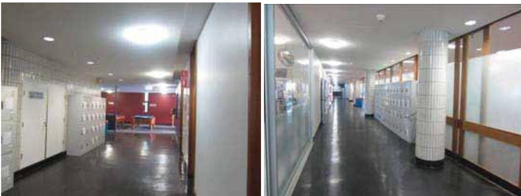
Figure 3-47 Spaces within the original section of Wentworth. Early fabric such as timber joinery and ceramic tile facings have survived.
