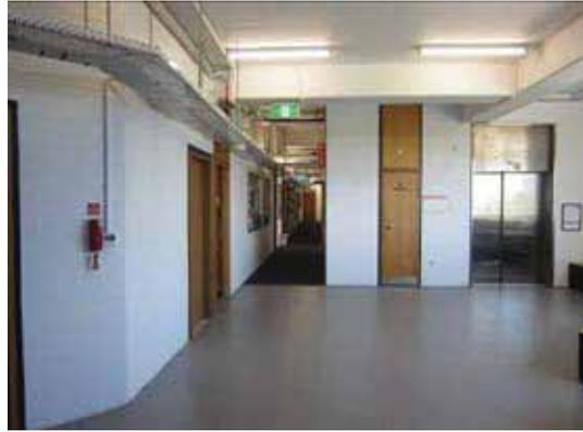
Figure 3-34 Upper level corridors and lift foyers have retained more early fabric, such as doors and brick walls. However, brickwork has been painted and intrusive new services introduced. Source: TKD Architects.
