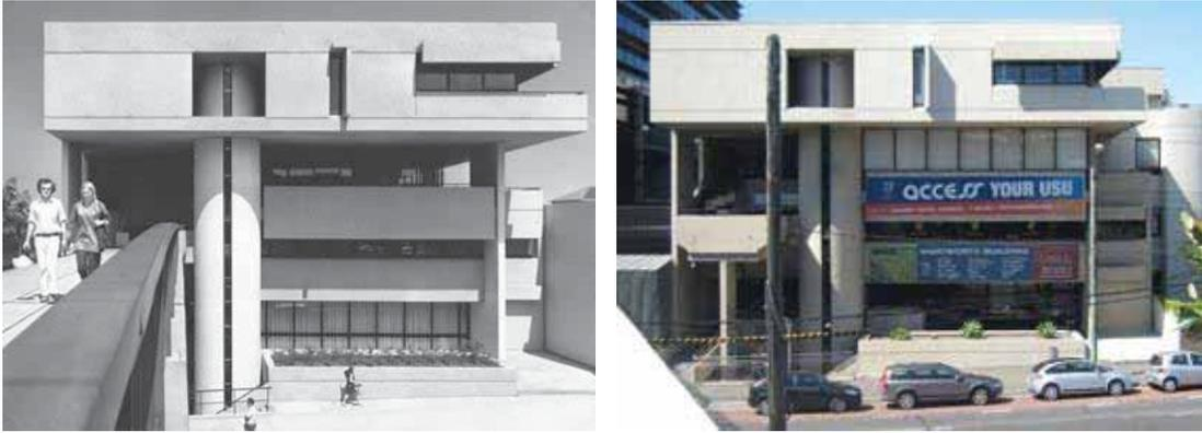
Figure 3-39 The character of the original City Road facade of the original component of the Wentworth Building is still very much in evidence, despite the relocation of the pedestrian bridge across City Road and the application of a coating to off-form concrete and ceramic tile finishes. Sources: National Archives Image No B4498, 29A5; TKD Architects.
