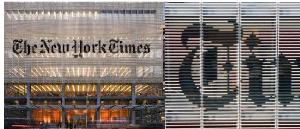
Example of building specific integrated signage, New York Times Building, New York
