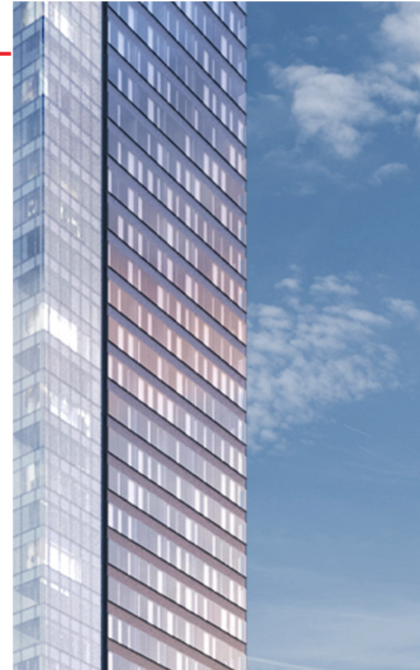
Detail view of main tower facade system
