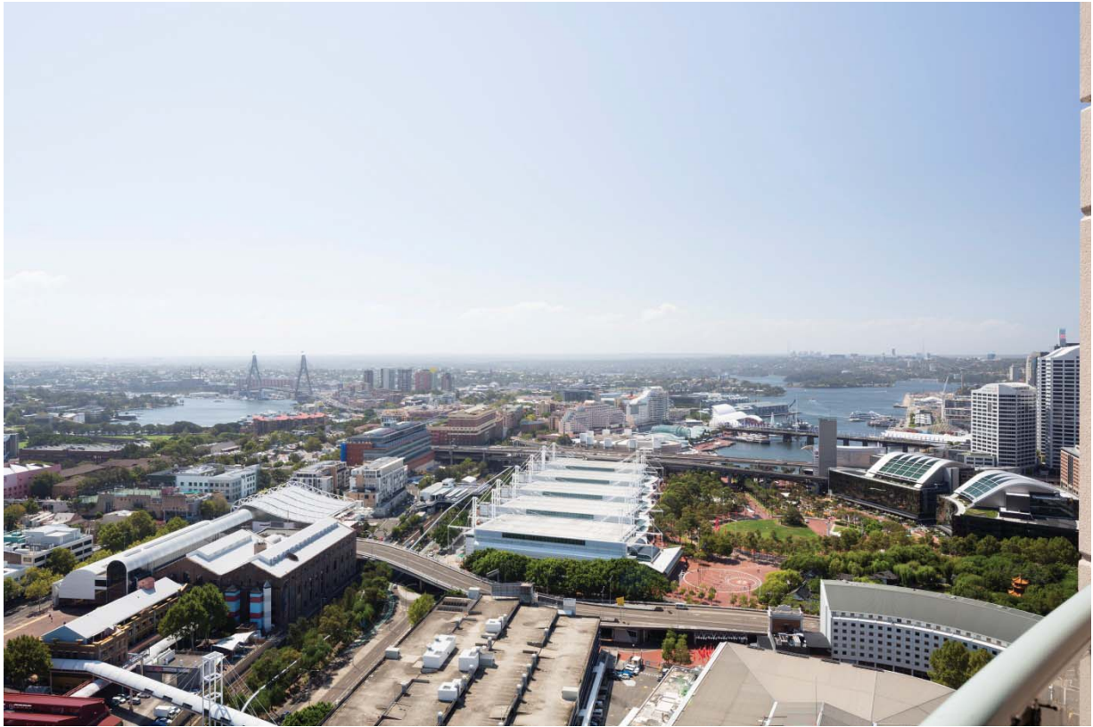
SICEEP-Peak Apartments 4209 EXISTING
