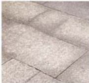
TIER 1 (PV04) - PEDESTRIAN CIRCULATION LARGE FORMAT PAVING
