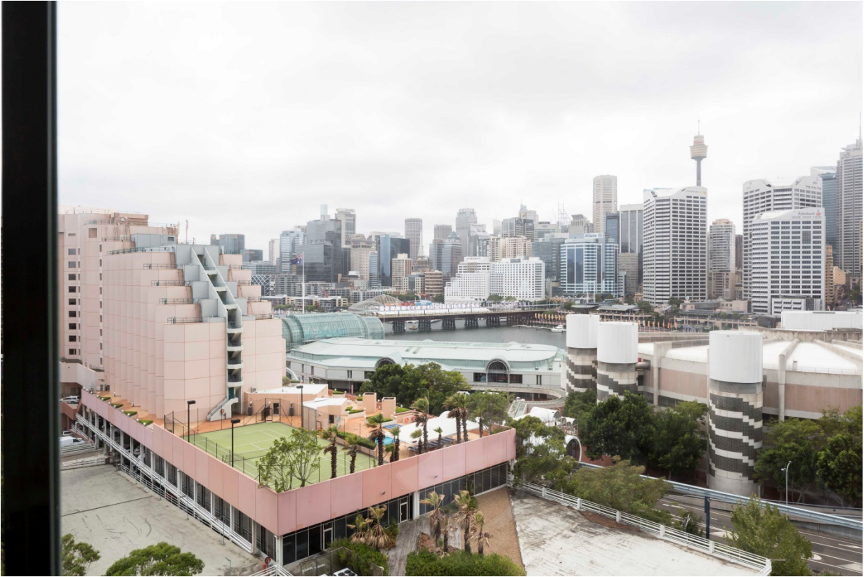
SICEEP-Goldsbrough 959 E EXISTING
