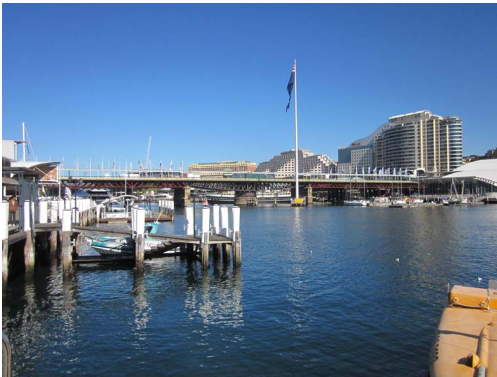
Figure 14 Setting of Pyrmont Bridge on the western side of Darling Harbour
