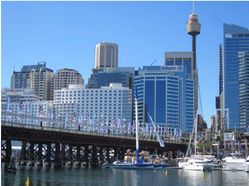
Figure 13 Setting of Pyrmont Bridge on the eastern side of Darling Harbour.
