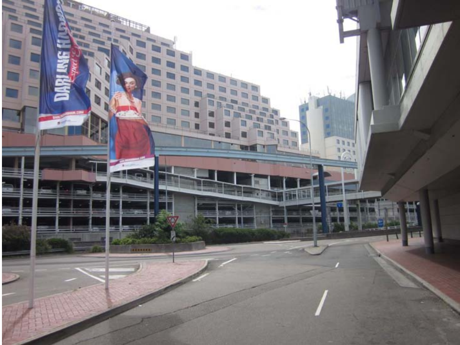
Figure 21 The Novotel and Harbourside Car Park viewed from the ICC Hotel site.
