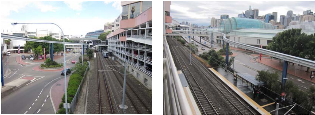
Darling Harbour Rail Corridor in the vicinity of the ICC Hotel site.
