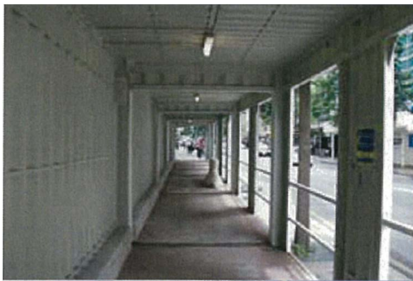
Figure 10 – Example of Class “B” Hoarding
