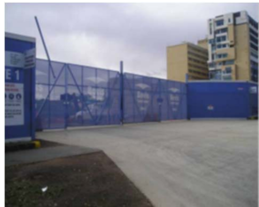
Figure 12 – Example of Class B Hoarding and Vehicle Entry Gates
