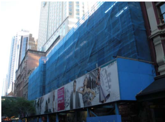
Figure 12 – Example of Class B Hoarding and Vehicle Entry Gates
