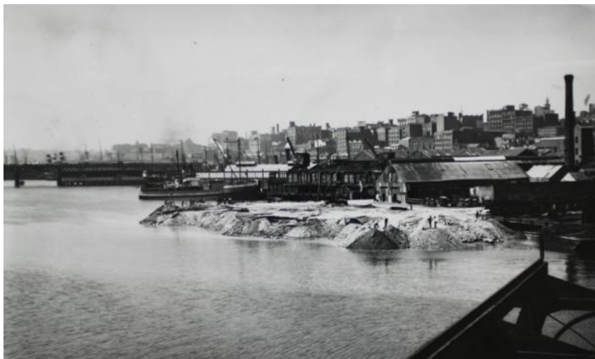
Figure 2.16: Fill from the Sydney railway construction dumped on the east shore of Darling harbour. NRS 17420 Item 848/15 SRNSW.
