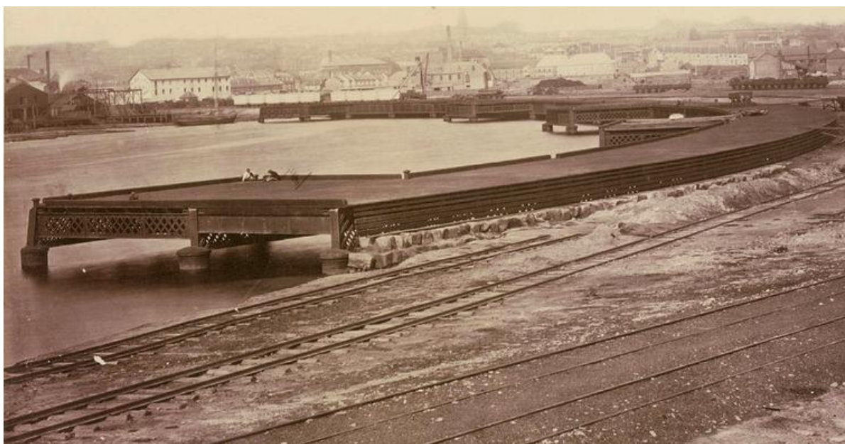
Figure 2.13: Undated photograph of the Iron Wharf, looking southeast. The stone seawall is visible behind the wharf and the fill almost complete suggesting a date of c1876. SLNSW SPF 844, digital order no. a089844.
