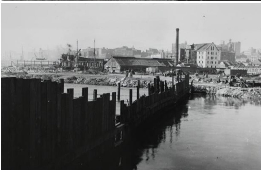
Figure 2.17: Fill extending along the east and southern shore of Darling Harbour and a wall of timber shoring built to temporarily retain the fill. NRS 17420 Item 848/16 SRNSW.
