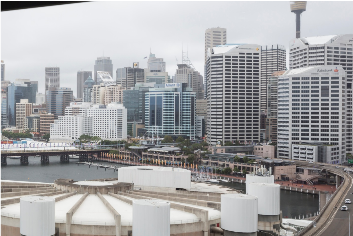
SICEEP-Goldsbrough 1303 E EXISTING
