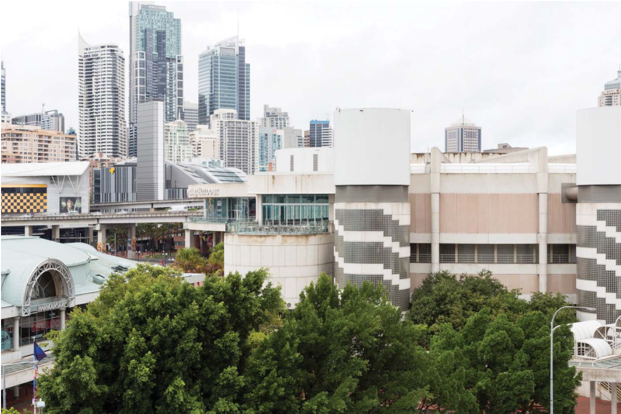
SICEEP-Novotel Deck 2 EXISTING
