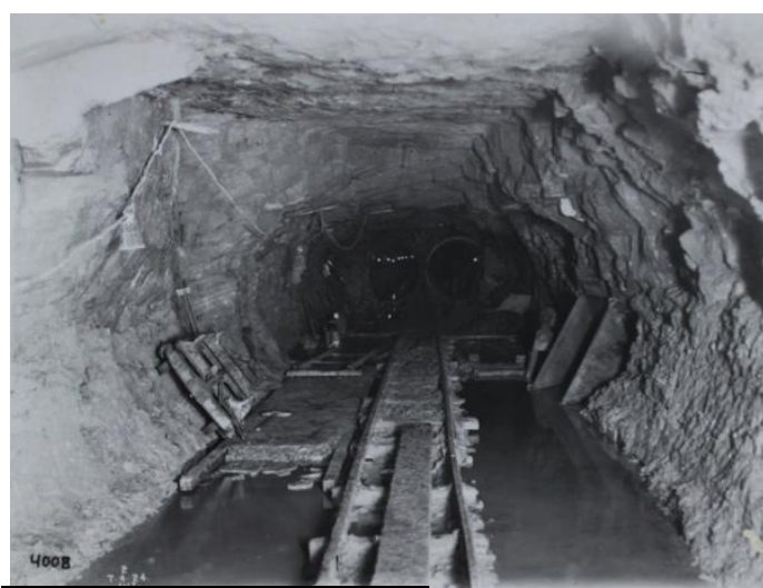
Figure 2.32: Excavation under Darling Harbour for the installation of water conduits for Ultimo Power House. State Rail Photos Series: 17420 Item: 364/44 SRNSW.
