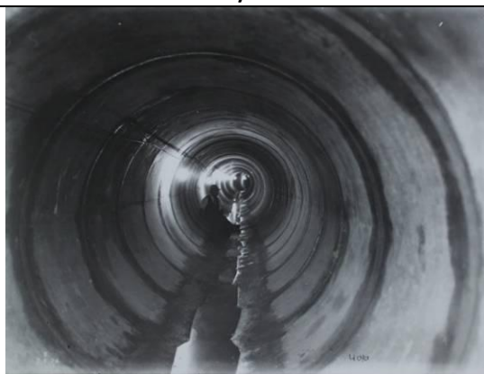
Figure 2.35: Joints between the sections of conduit are visible along the length of the water supply pipe. State Rail Photos Series: 17420 Item: 364/47 SRNSW.
