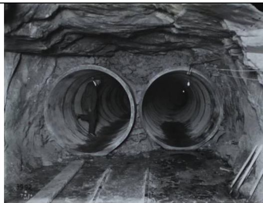
Figure 2.34: Rails in the foreground were used to cart rubble fill to the pipes. State Rail Photos Series: 17420 Item: 364/46 SRNSW.
