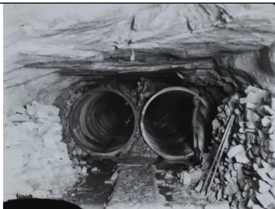
Figure 2.33: Pair of RC Monier conduits being installed in the sandstone tunnel under Darling Harbour. Rubble is stacked ready for packing around the 6 ft diameter pipes. State Rail Photos Series: 17420 Item: 364/45 SRNSW.
