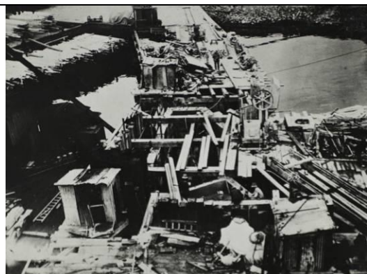
Figure 2.36: Cofferdam and formwork for the installation of conduits. State Rail Photos Series: 17420 Item: 364/48A SRNSW.
