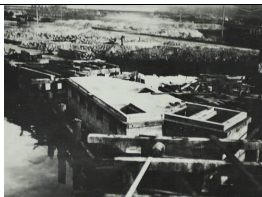
Figure 2.38: Work undertaken at the water's edge for installation of the inlet conduits for the Ultimo Power House. State Rail Photo Series: 17420 Item: 364/48C SRNSW.
