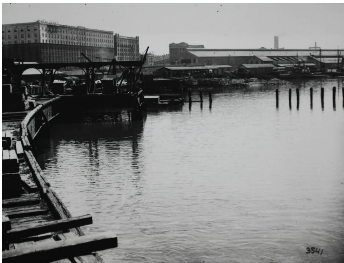
Figure 2.29: A photograph looking northwest at the Iron Wharf, Darling Harbour, c1920, at the beginning of demolition work. NRS 17420 Item 848/18 SRNSW.
