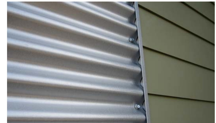
typical profiled metal sheeting
