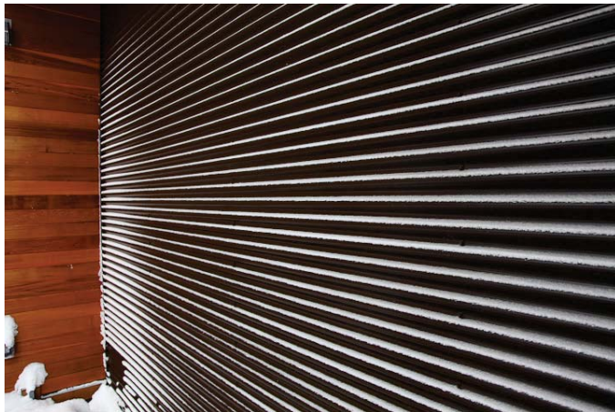
typical profiled metal sheeting (horizontal)
