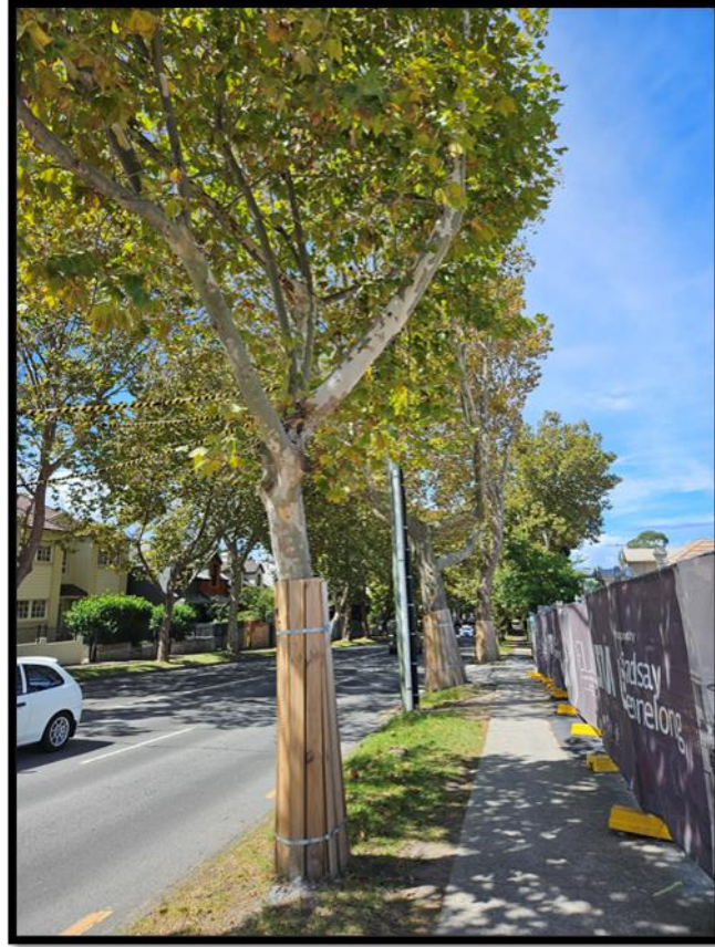
Figure 8 - Example of stem protection boarding required on all retained trees within the site.
