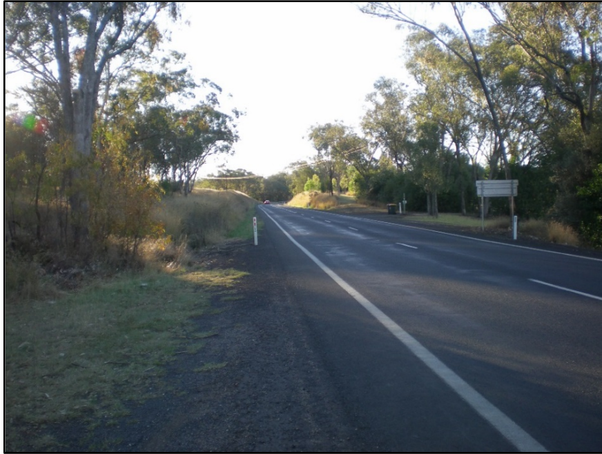
■ Photo 8 Example of non-conforming sealed shoulders on Gwydir Highway approximately 1km west of Bindaree Beef site
