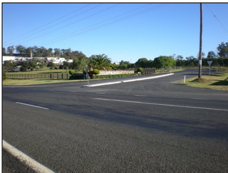
■ Photo 1 Access Point 1 - All traffic non-emergency traffic between Gwydir Highway and Bindaree Beef site must use this access point
