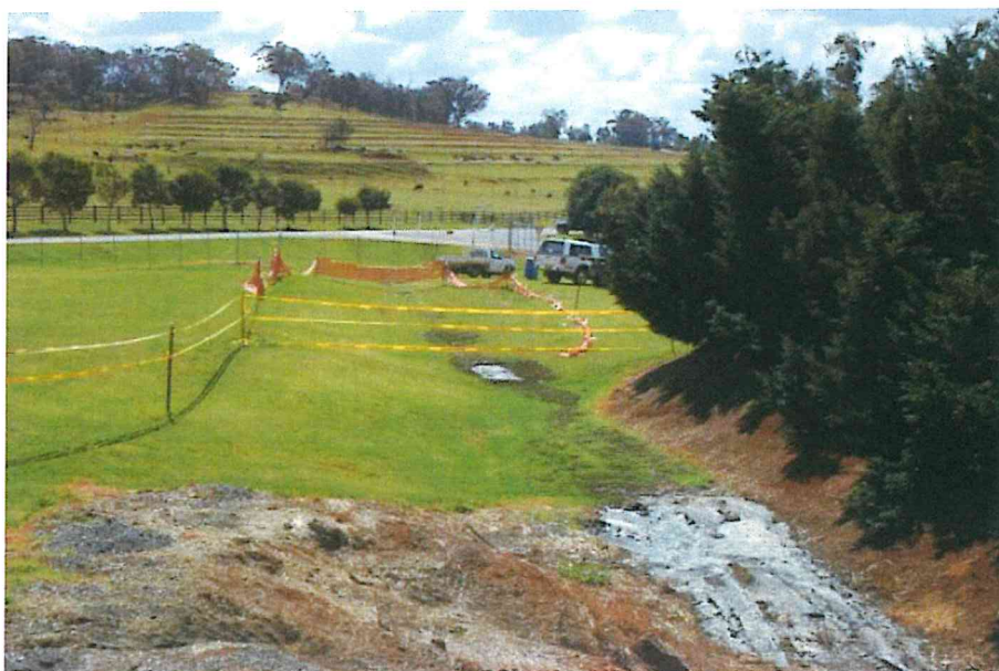
Figure 12 Swale Drain (view from plant)
