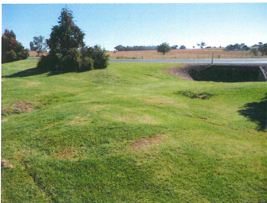
Figure 13 Existing Culvert at Highway (view looking northwest)
