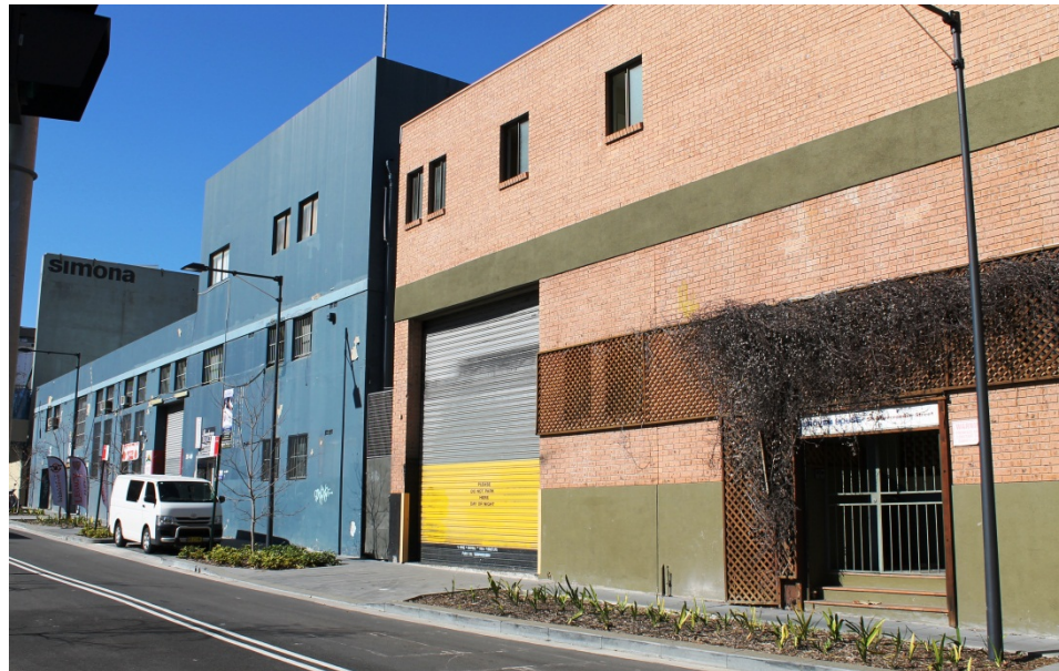
Figure 5 – Commercial development along O'Connor Street
