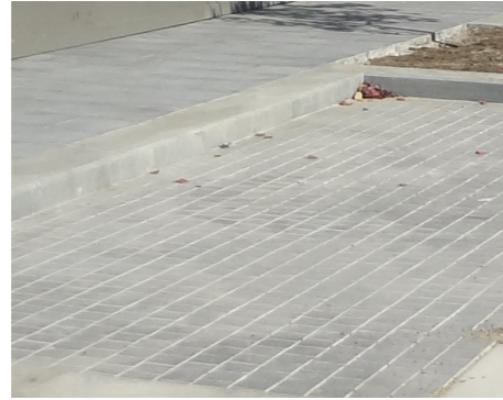
O'Connor Street Parking Bay
