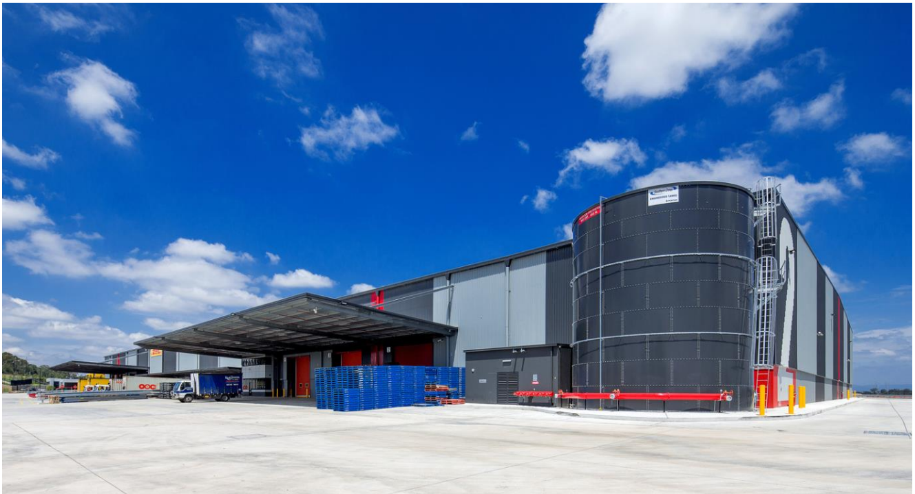
Figure 1 - Existing water tank at Oakdale Central
