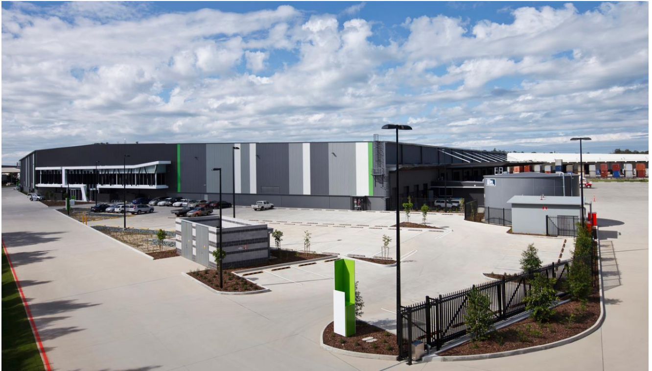
Figure 2 - Lytton Motorway Estate, Queensland
