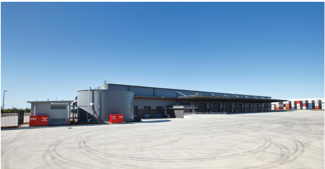
Figure 3 - Lytton Motorway Estate, Queensland
