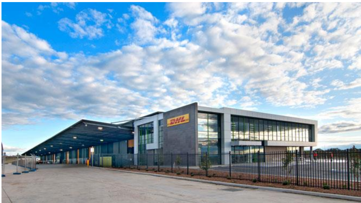
Figure 3: Recently constructed DHL warehouse within Oakdale Central
