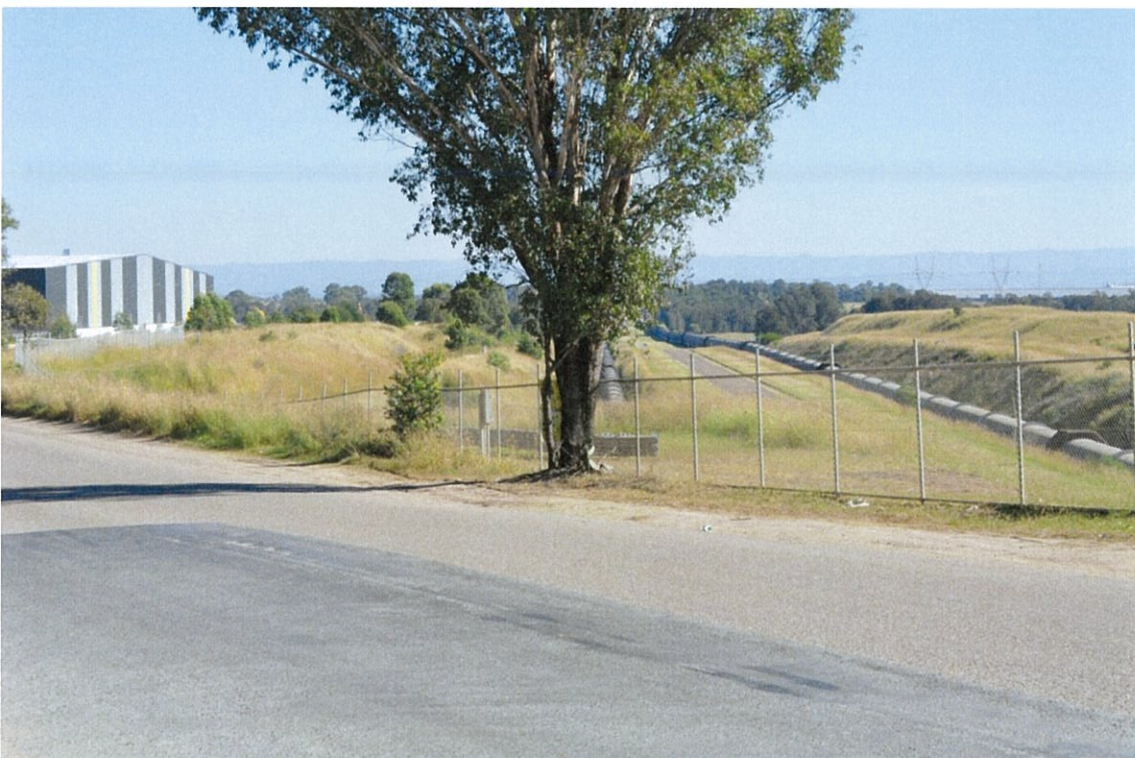
Figure 3.6 View D. Extensive excavations and soil build up to traverse the Sydney Water Supply pipelines. (Source: GML 2014)
