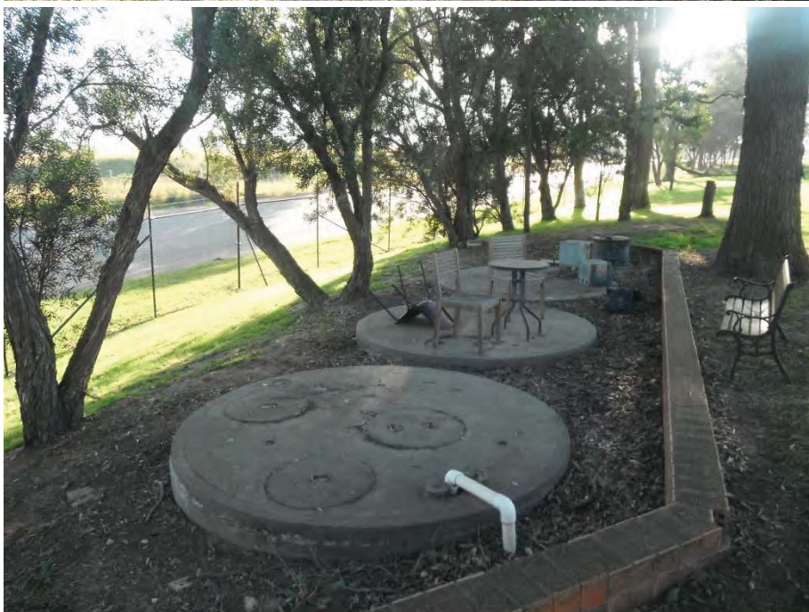
Plate 4: 3 x septic tanks, Austral Bricks. Treated effluent is used for lawn irrigation.
