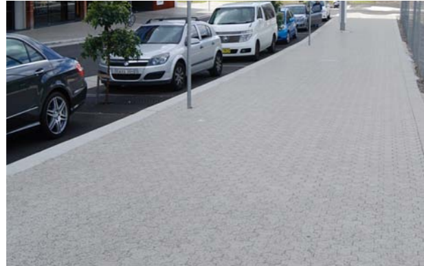
TRIHEx PAVING TO MATCH EXISTING (P9)
