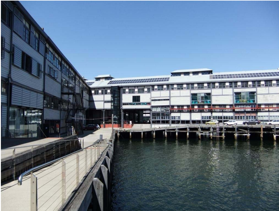
Photo 1: View looking south-west with shore sheds to the left of photo and Wharf 4/5 to the right.
