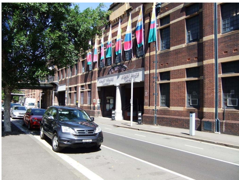
Photo 6: Shore sheds along Hickson Road showing entry to Wharf 4/5
