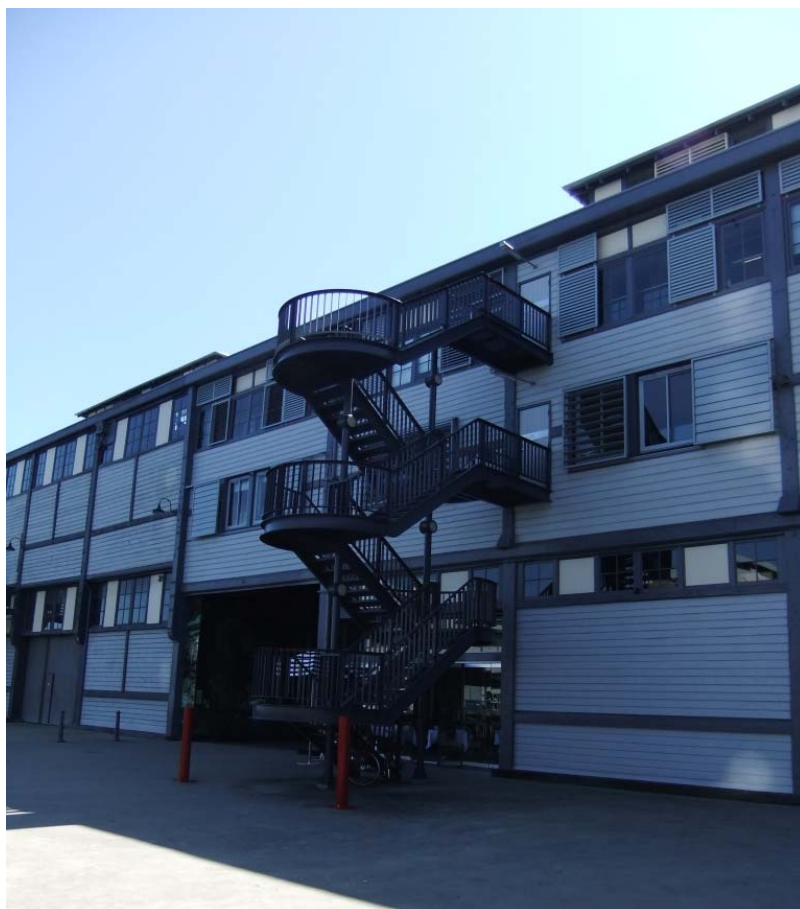
Photo 4: Existing offices in Pier 2/3
