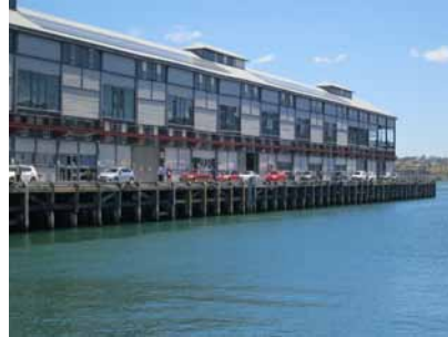
Figure 2.5.4: Wharf 4/5 east elevation
