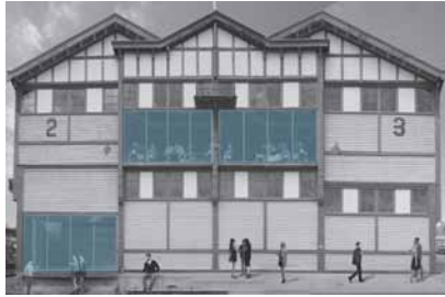
Figure 7.4.2: Openings in the north end of Pier 2/3. Openings located in the middle of the elevation retain solidity at the corners. Potential for a new opening in on the east side of ground floor to interpret the original loggia (since filled in) and to address the asymmetry of the elevation.
