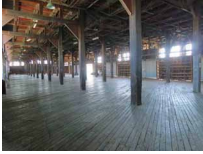
Figure 2.4.11: Pier 2/3 Ground floor, north end looking north
