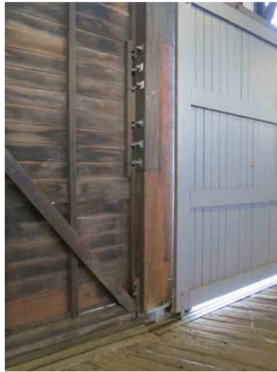
Figure 2.4.16: Pier 2/3 Ground floor, previous pier. Repair and splice.
