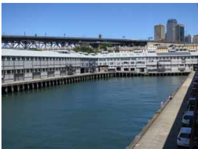
Figure 2.4.7: Aprons. From Wharf 4/5, looking south east towards shore shed and Pier 2/3.
