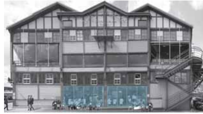
Figure 7.4.3: New openings in the north end of Wharf 4/5 on ground floor. Openings located in the middle of the elevation retain solidity of the ground floor corners.
