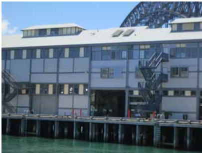
Figure 2.4.5: Pier 2/3 breezeway, west elevation
