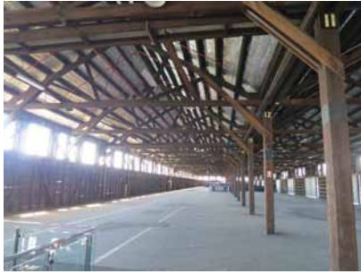
Figure 2.4.19: Pier 2/3 Upper deck, looking north
