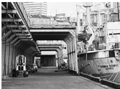
Figure 7.2.4: West elevation of Wharf 4/5, c1975, © Alan Croker
