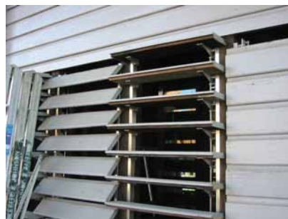
Figure 7.4.5: Jones Bay Wharf – use of weatherboards as operable tilted louvres.
