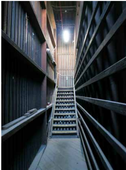
Figure 2.4.15: Pier 2/3 Ground floor, early fire tunnel
