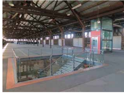
Figure 2.4.20: Pier 2/3 Upper deck lift and stair c.2003
