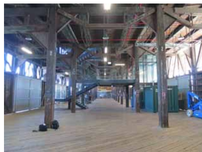
Figure 2.4.9: Pier 2/3, Ground floor, south end looking north. Stair and lift insertion c.2003. Note container in right of image containing moveable heritage from Towns Place.
