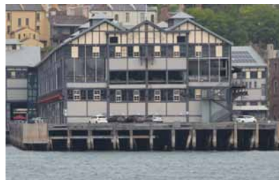
Figure 2.5.6: Wharf 4/5 north elevation (taken from McMahon's Point)
