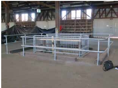
Figure 2.4.21: Pier 2/3 Upper deck, top of early fire stair. Handrails later additions.
