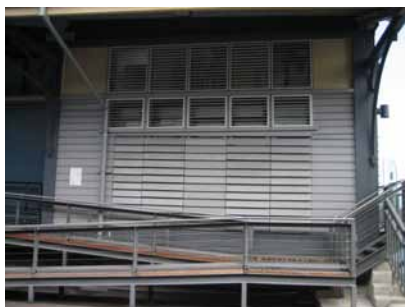
Figure 7.4.4: Jones Bay Wharf – use of weatherboards for operable tilted louvres retained solidity of the walls as solid wall when closed.
