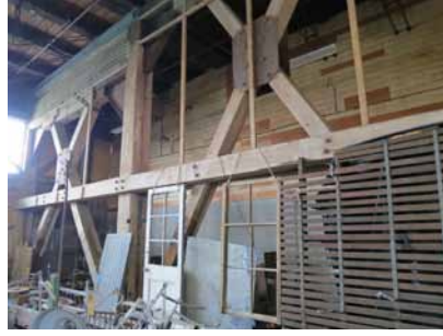
Figure 2.4.12: Pier 2/3 Ground floor, structural framing, former shower rooms.
