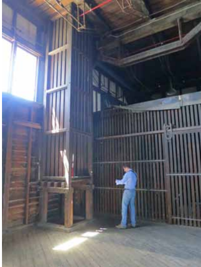
Figure 2.4.17: Pier 2/3 Ground floor bag chute.
