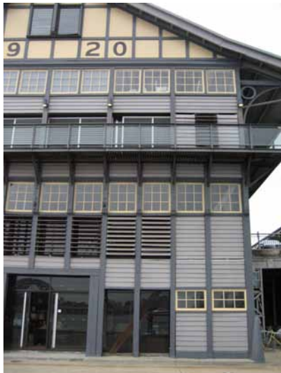
Figure 7.4.2: Jones Bay Wharf – use of weatherboards as tilted louvres shown in various forms of full open, half open and closed.
