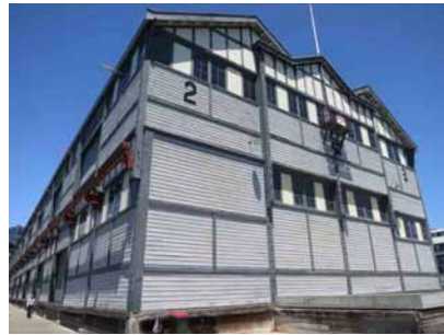
Figure 2.4.6: Pier 2/3 North Elevation
