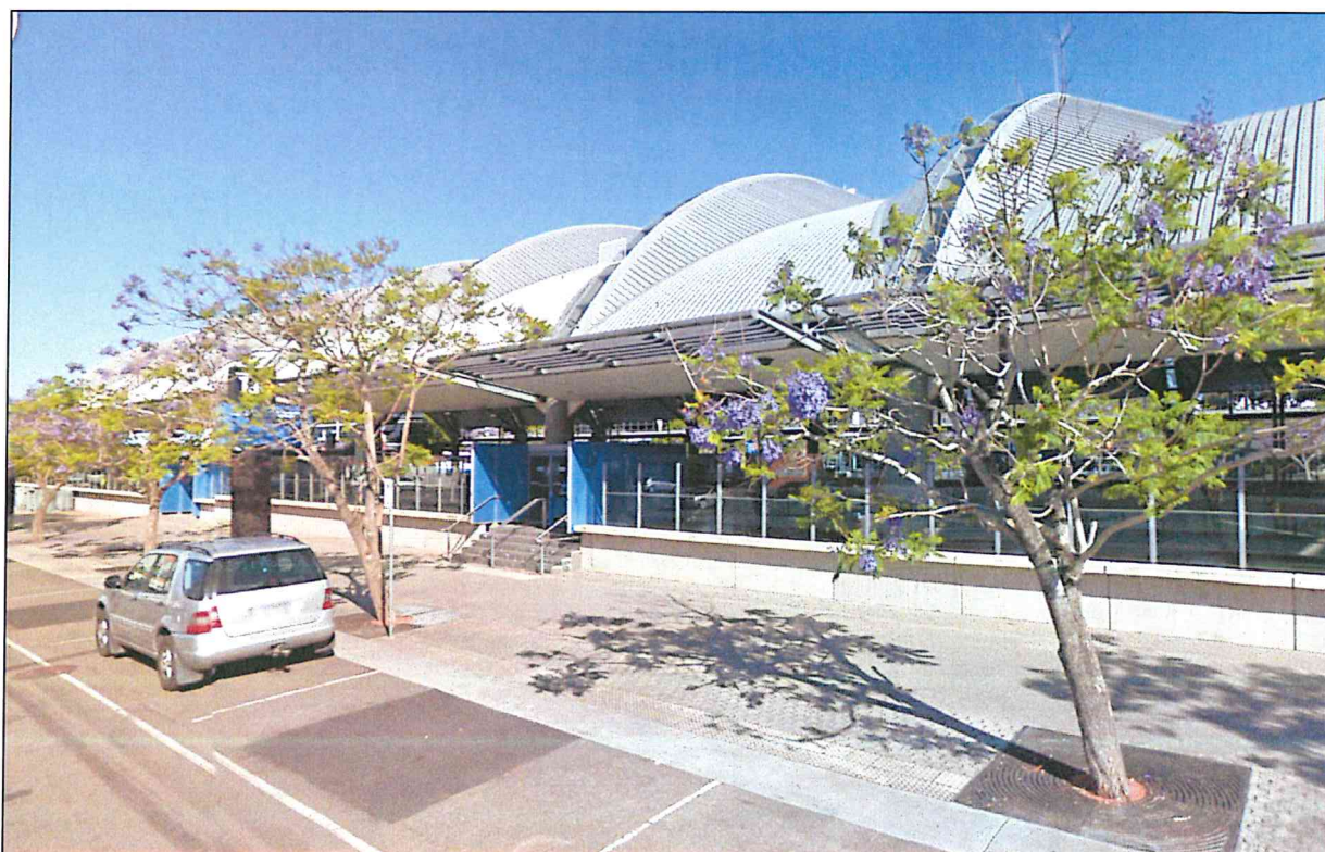
Figure 3: Olympic Park Railway Station
