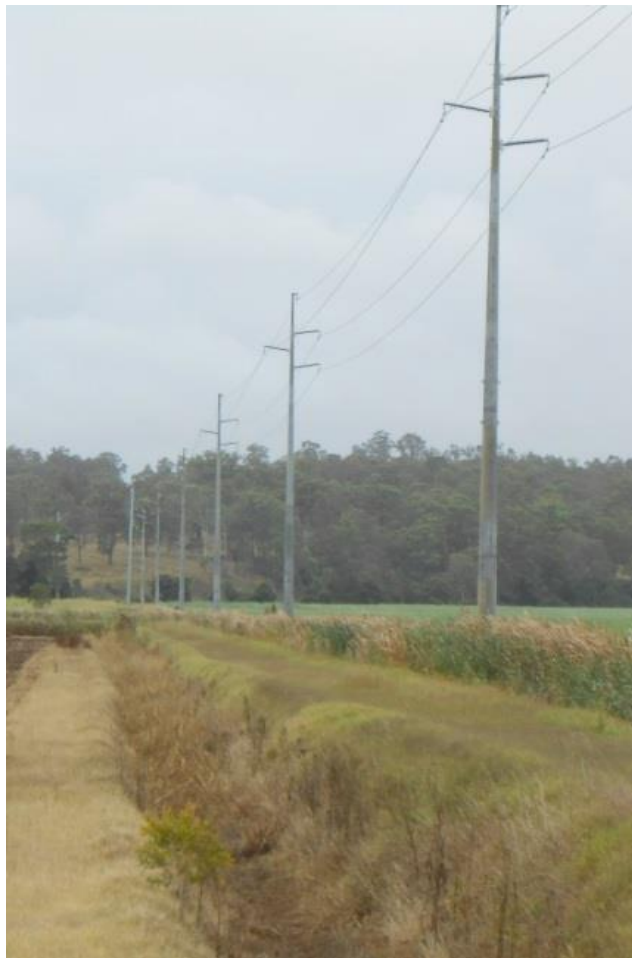
Figure 5.1 Proposed Biala 132 kV transmission line configuration
