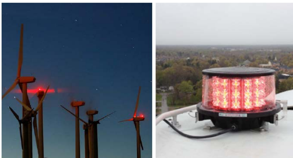
Photograph 3-1 Typical WTG Obstacle Lighting (Source: Clouston Associates 2015)
