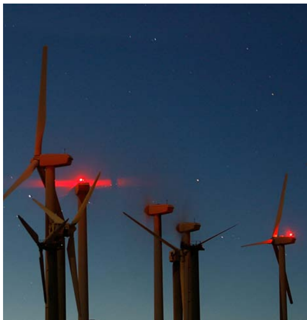
Typical WTG obstacle light
