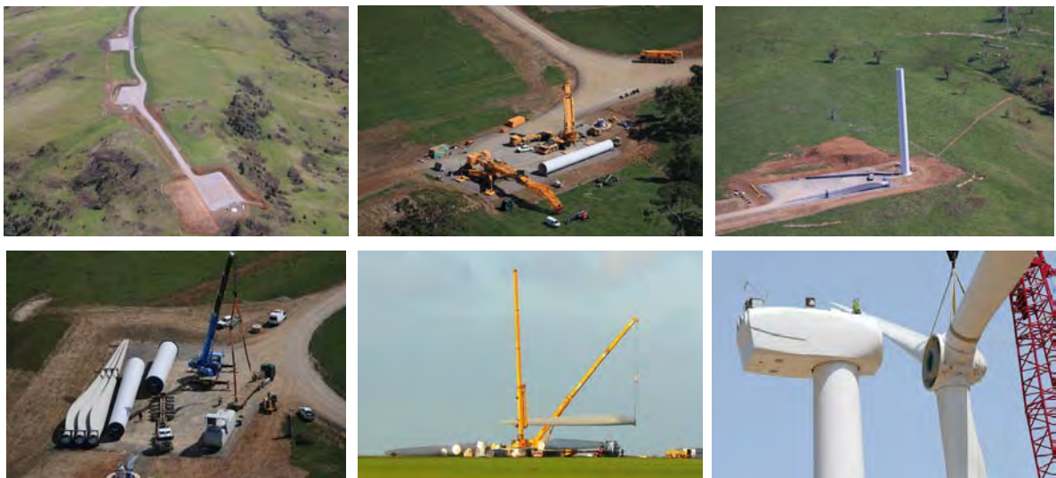
Typical construction activity
