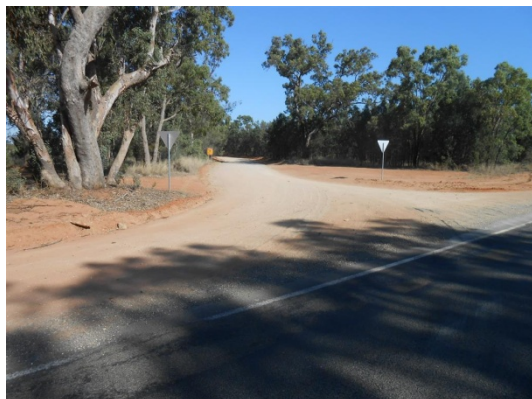
Figure 2.7: Westport Road at the Newell Highway
