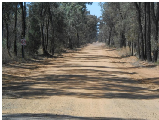
Figure 2.6: X-line Road (looking east)
