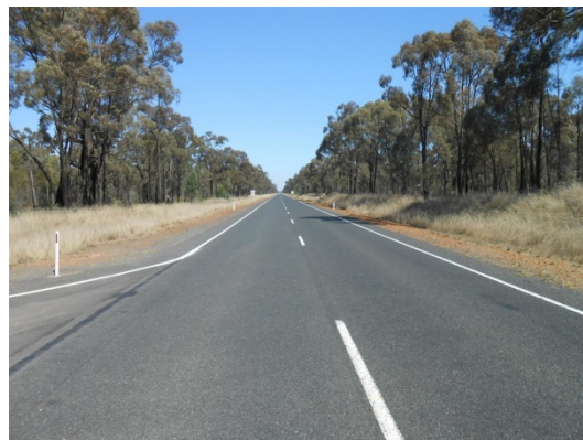
Figure 2.4: The Newell Highway (looking south from X-line Road)
