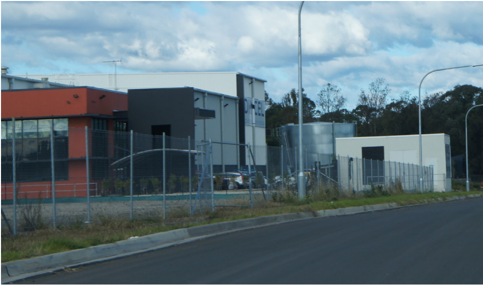
View of 101 Quarry Road (from the north)
