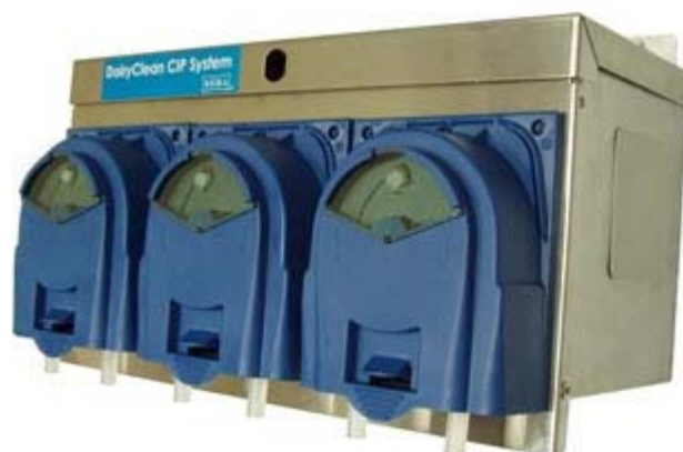
Figure 5-3: Example of CIP Dispensing Pump System (DEMA 2013)
