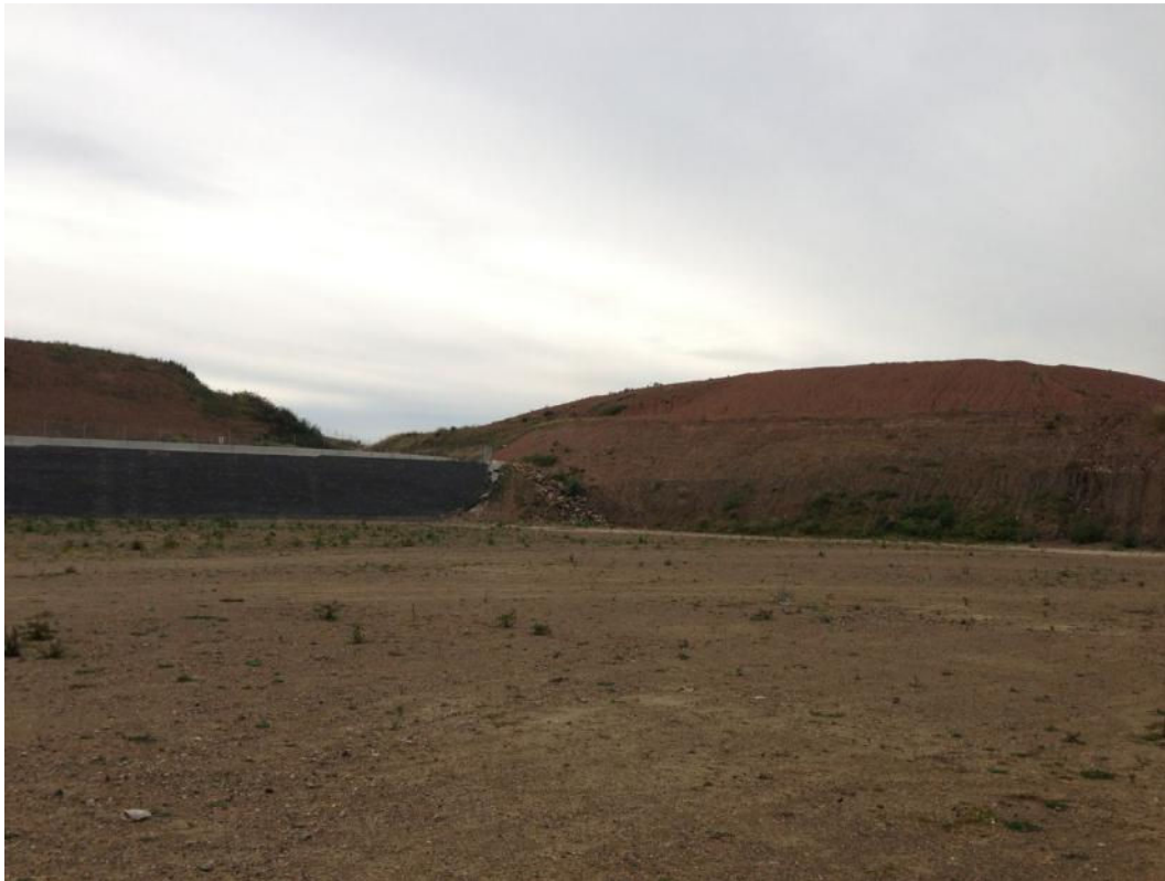
Figure 1 View to northeast showing the northern boundary retaining wall and eastern fill embankments
