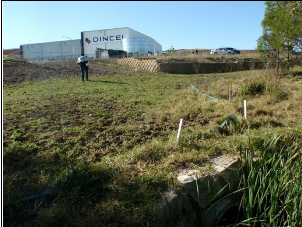
13u – view to north from pipe outlet showing upstream drainage catchment
