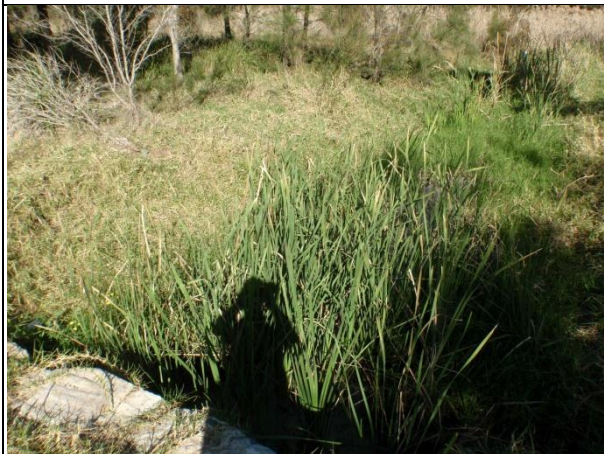
13d – view to south along flowline of stormwater outlet, headwall in bottom left corner
