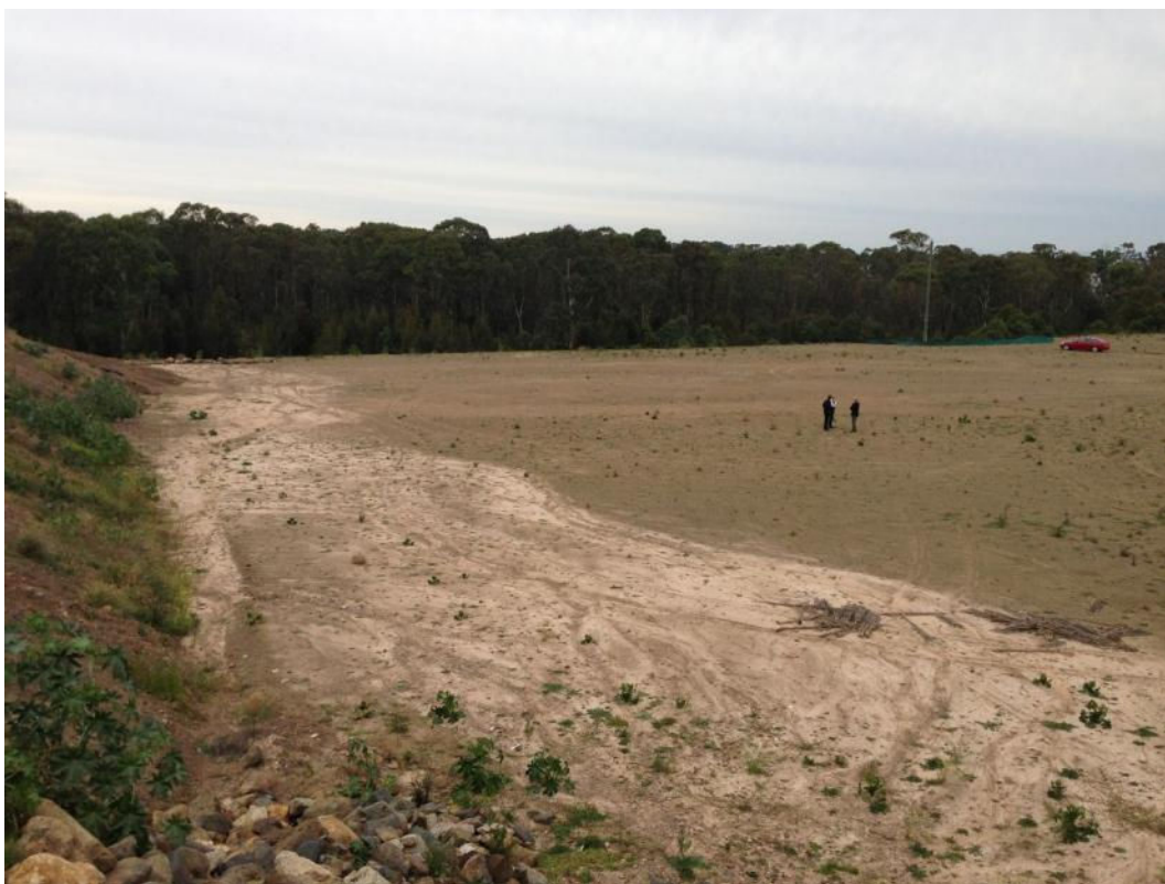
Figure 2 View to the south along the eastern boundary showing sediment deposition from upslope runoff
