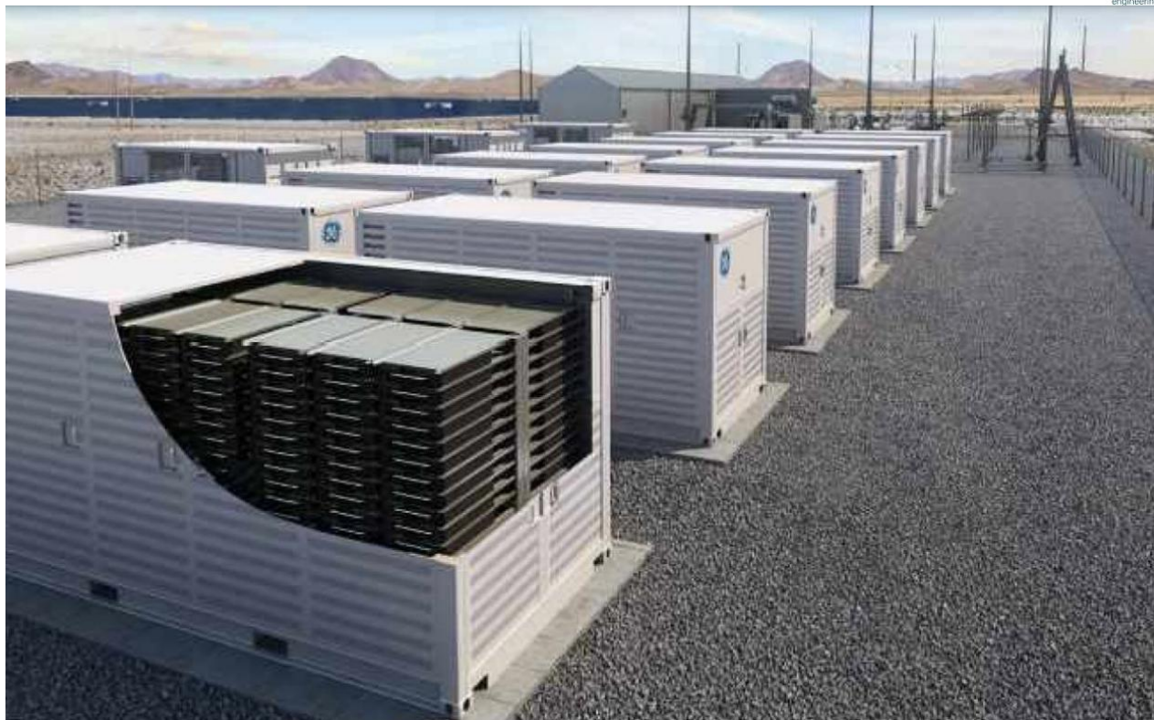
Figure 3-8: BESS exemplar arrangement
