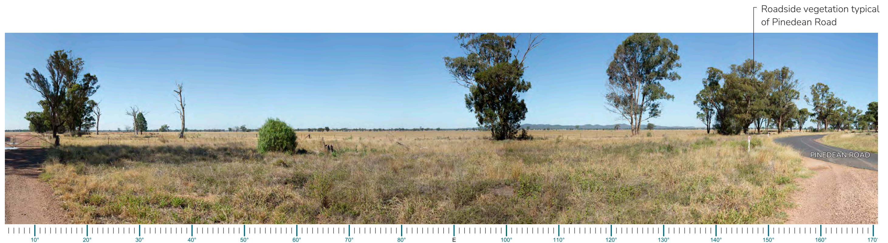
Figure 34 Existing View from corner of Pinedean Road looking in an east direction. The proposed 132kV Transmission Line runs parallel to Pinedean Road for approximately 1,370 m
