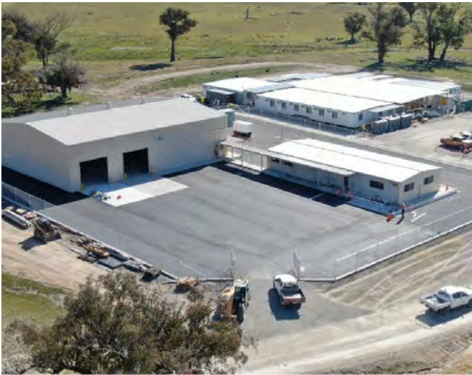
Image 03 Typical O&M Facility (Source: ERM)
