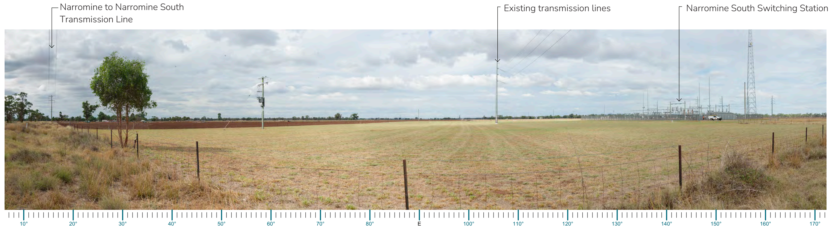
Figure 33 Existing View from Gainsborough Road, looking East towards the Narrabri Substation
