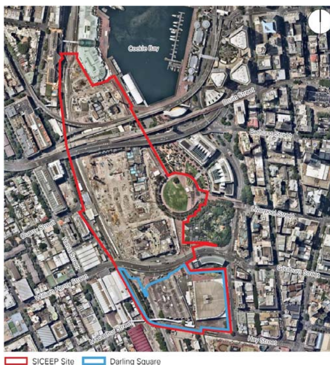
Figure 1 – Aerial Photograph of the SICEEP Site
