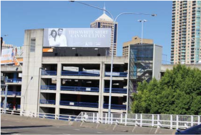
G. View from Pier St roadway
