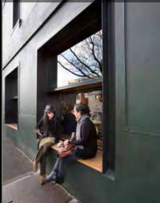
Seating elements into façade
