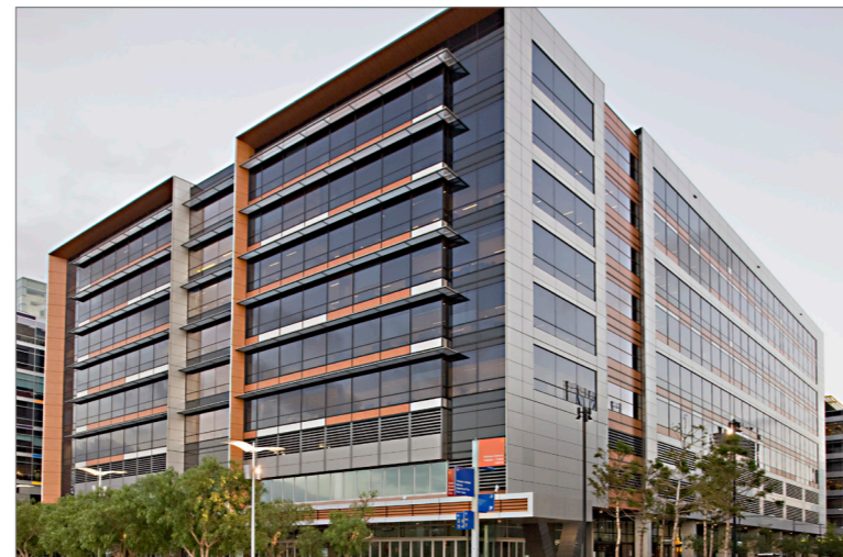
FACADE BENCHMARK - ERICSSON, MELBOURNE
