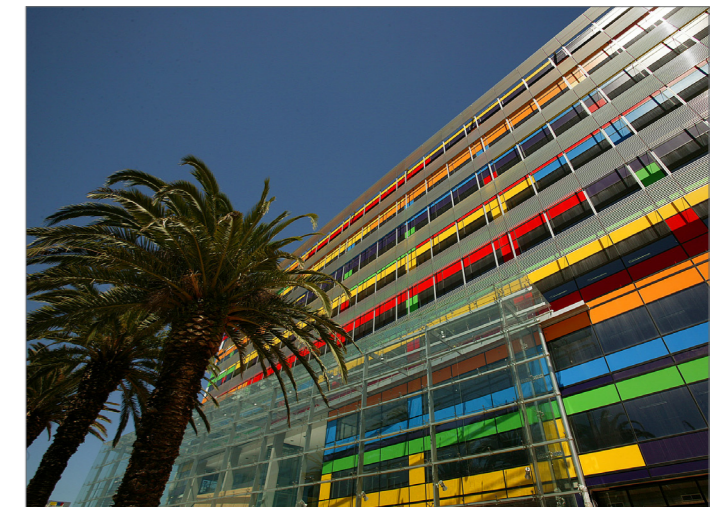
FACADE BENCHMARK - NAB, MELBOURNE
