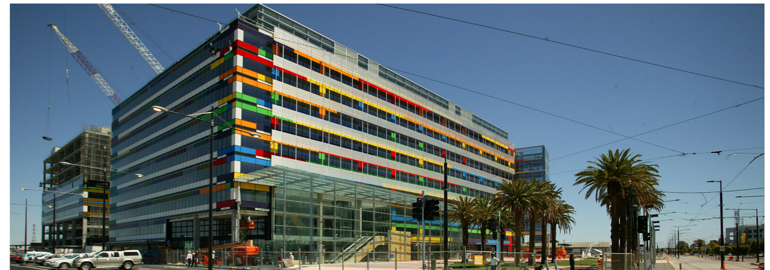
BENCHMARK PROJECT - NAB, MELBOURNE
