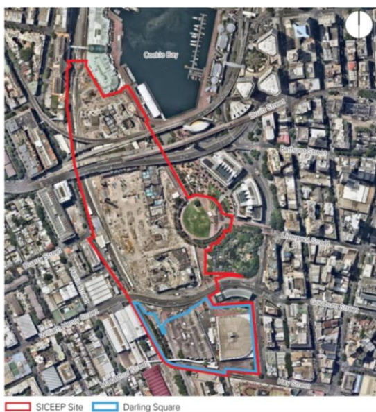
Figure 1 – Aerial Photograph of the SICEEP Site
