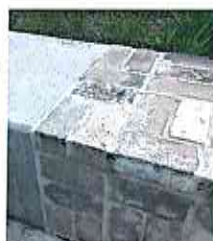
Recycled brick wall
