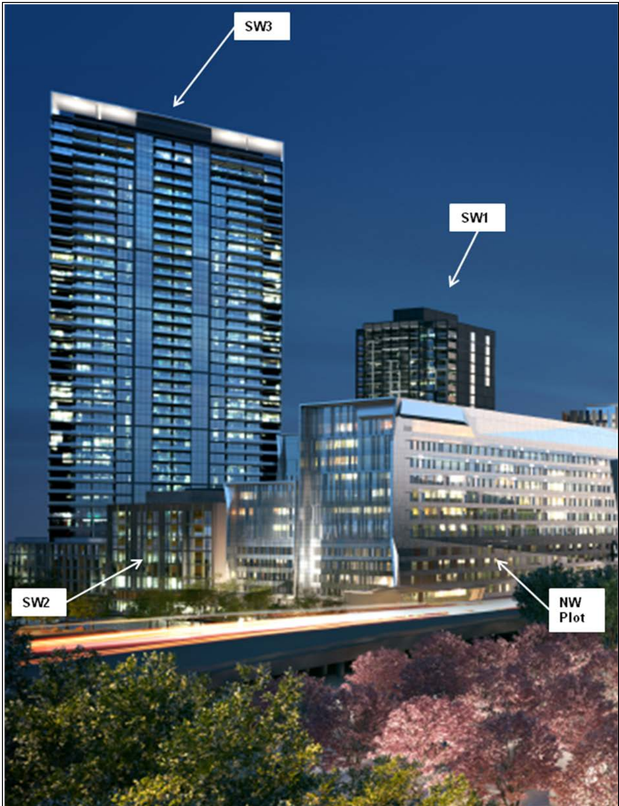
Figure 8: View south west to the South West Plot and North West Plot across the Pier Street overpass (Base source: applicant's RtS)
