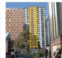
Macarthur street view with projecting apartment highlighted
