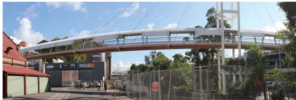
EXISTING CONDITIONS VIEW NORTH
