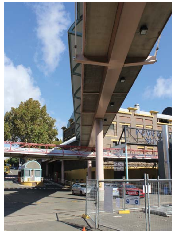
EXISTING CONDITIONS VIEW WEST
