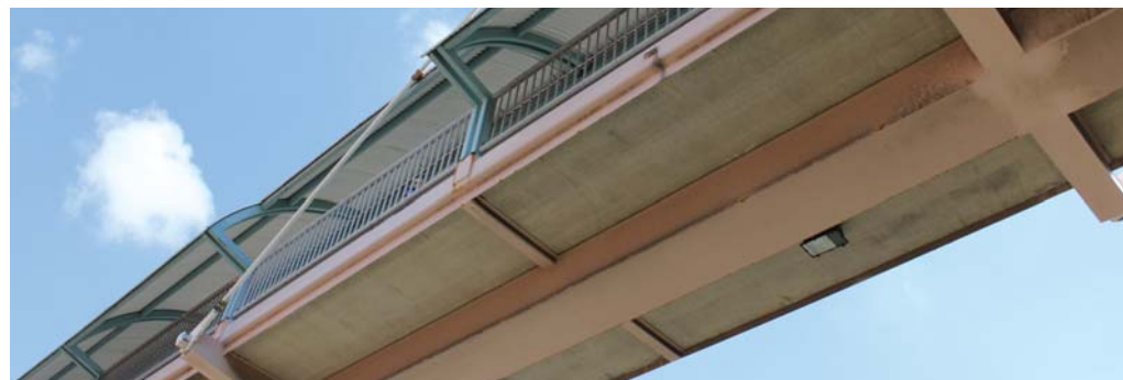
EXISTING CONDITIONS DETAIL VIEW OF UNDERSIDE
