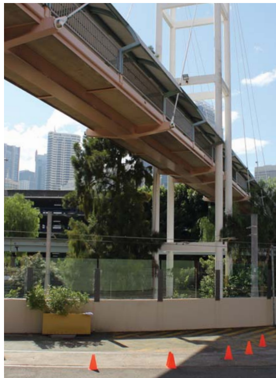
EXISTING CONDITIONS VIEW EAST
