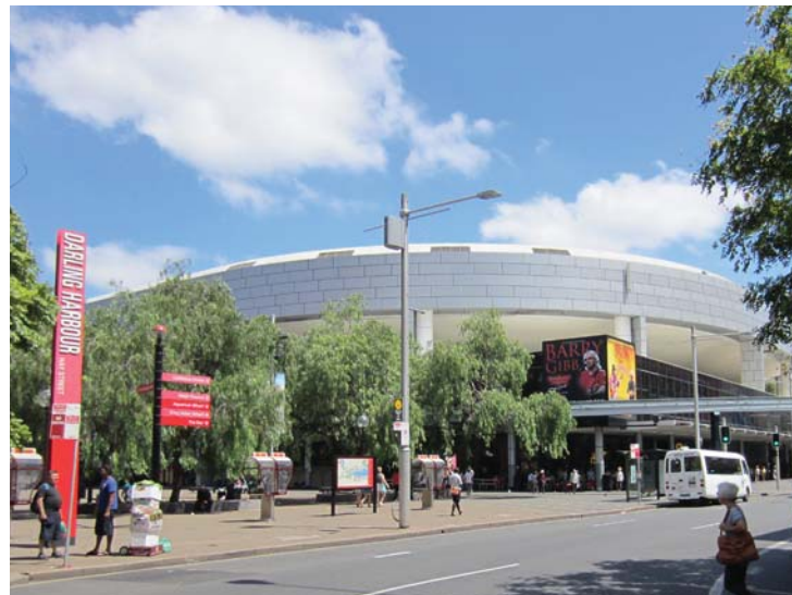
Existing Entertainment Centre
