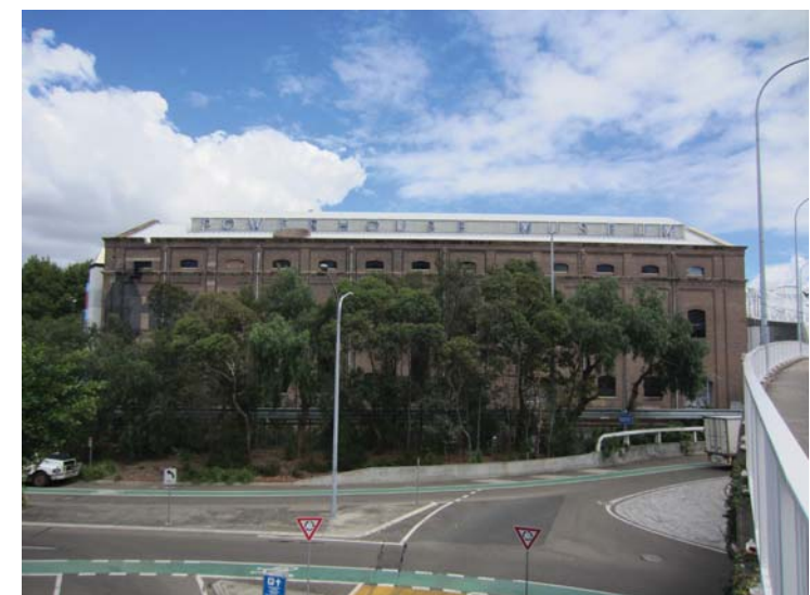
Heritage Pumpphouse building
