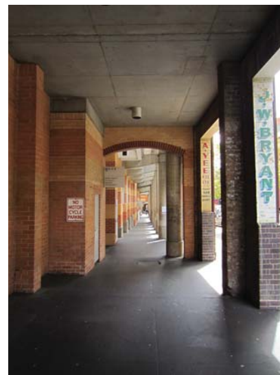
Colonnade along Quay Street (looking north)
