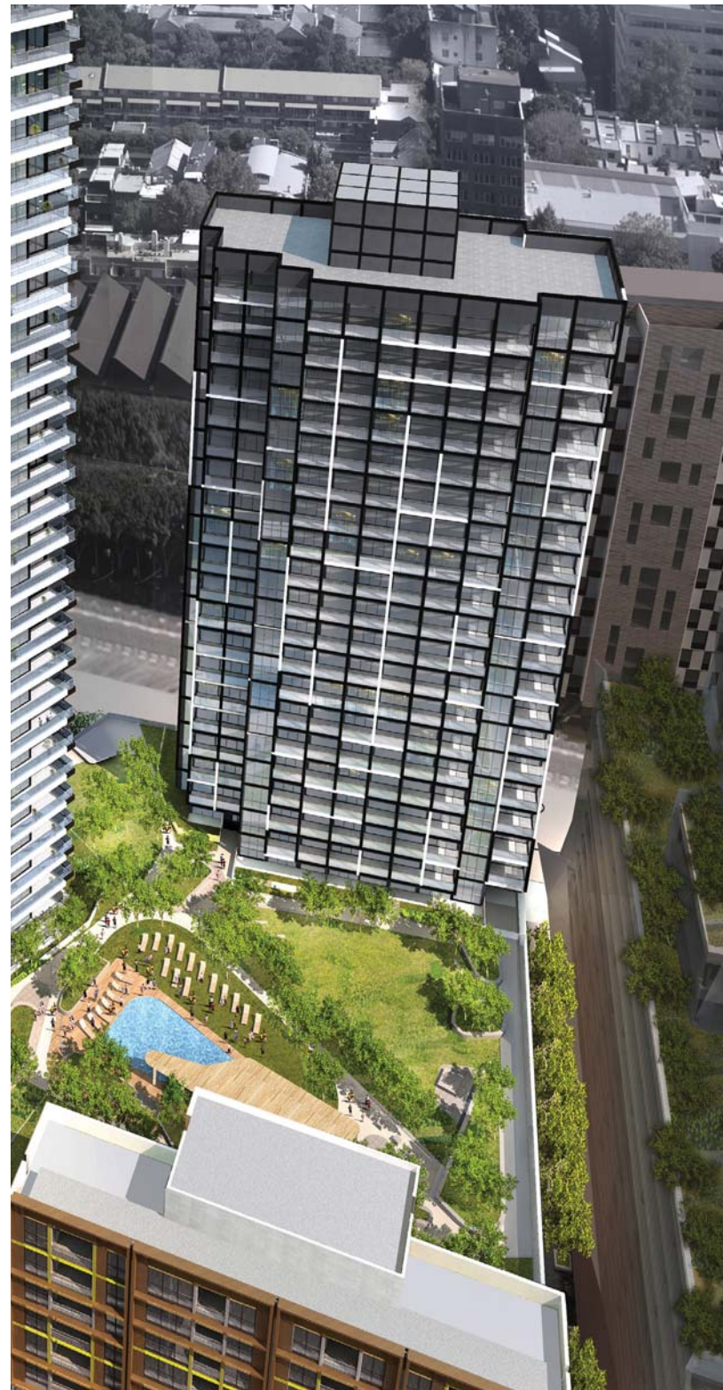
SW1 Tower viewed from east
