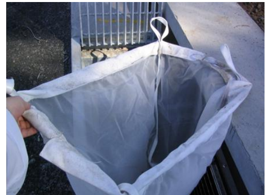
Figure 10 A typical Enviropod pit insert assembly (Source: Stormwater360)
