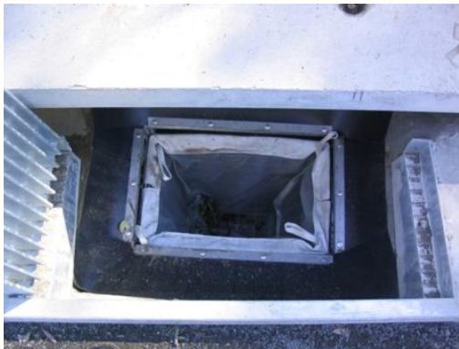
Figure 10 A typical Enviropod pit insert assembly (Source: Stormwater360)
