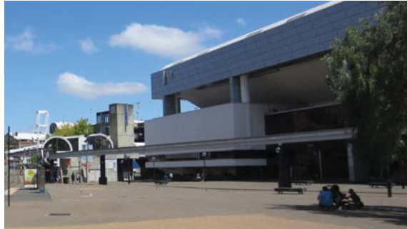
Existing Hay Street looking east
