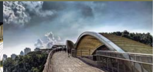
ELEVATED TIMBER DECK THROUGH THE CANOPY
