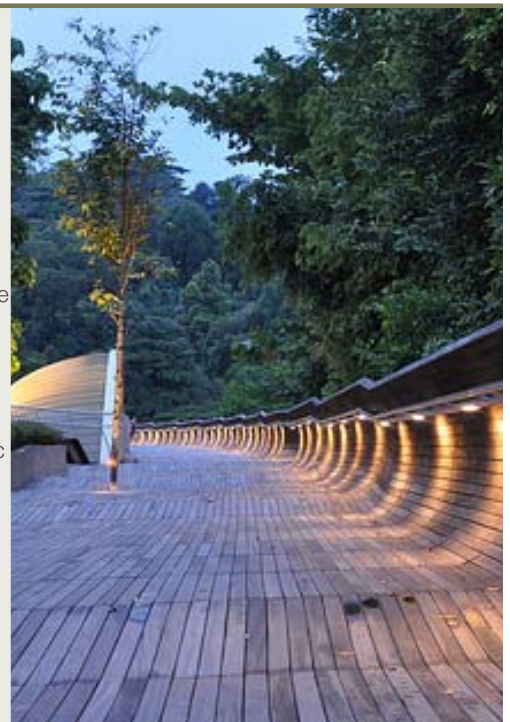
GARDEN CITY PEDESTRIAN BRIDGE, SINGAPORE
