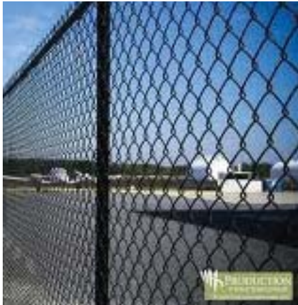
Figure 14 Security fence- PVC coated chain mesh
