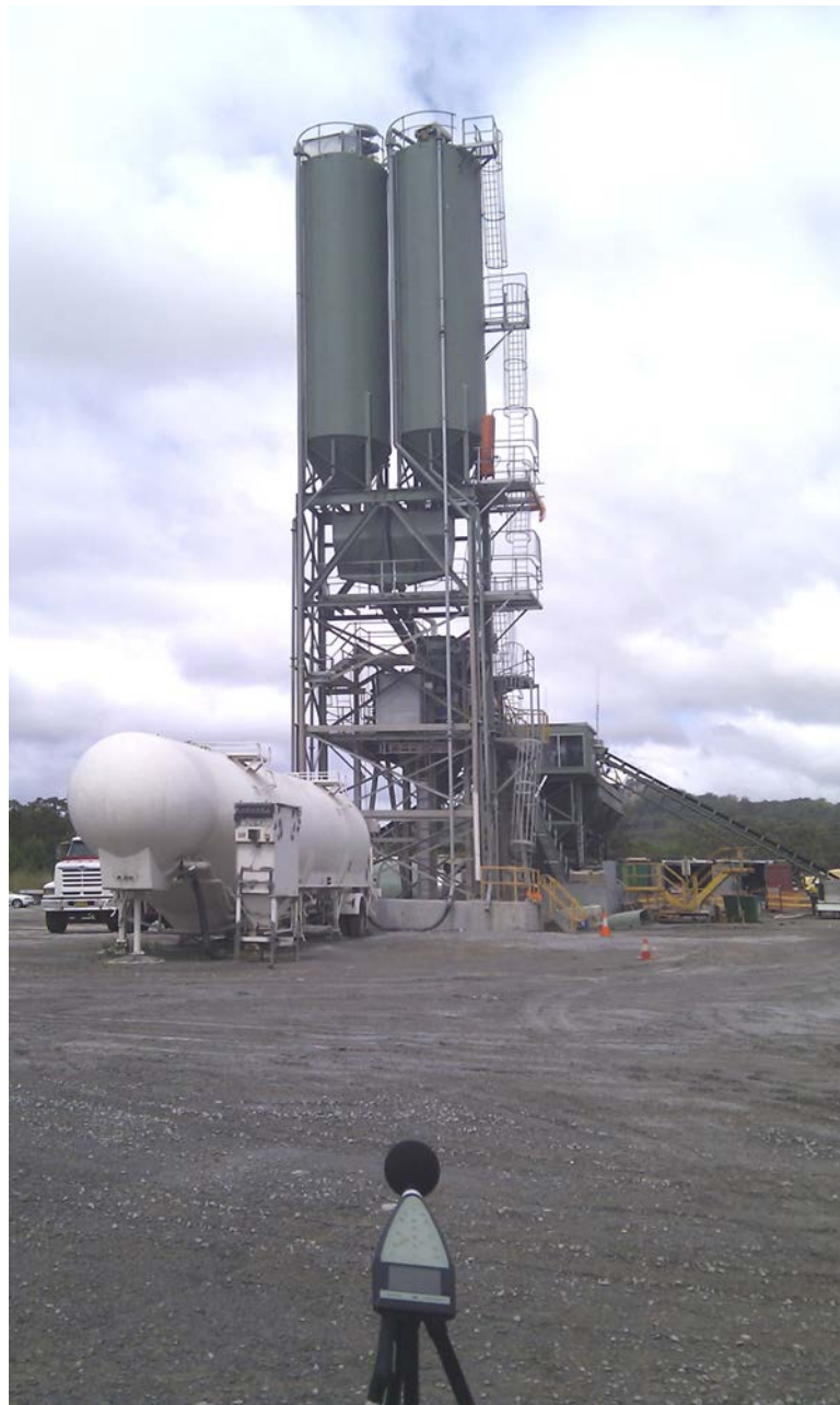
Figure 4-1 Concrete Batch Plant
